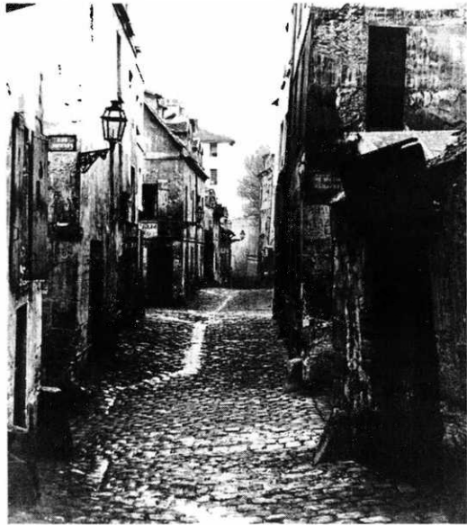
Paris before Haussmann: Charles Marville's photograph of the Rue Traversine. Notice the drainage ditch in the center of the cobblestone street.
