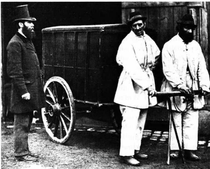
Street disinfectors in London, 1875.
